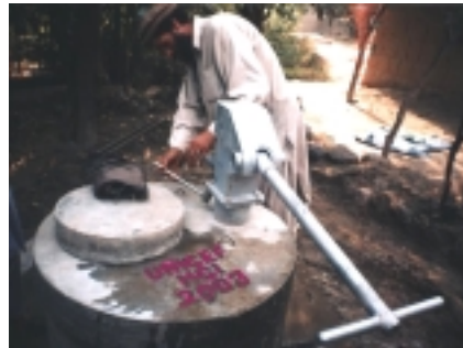
Another water project in Afghanistan
